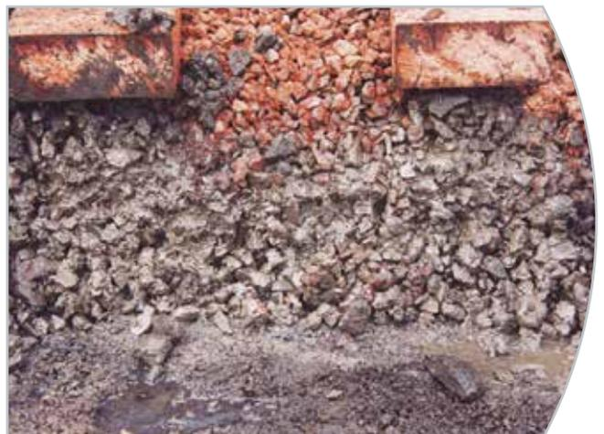
Severe subgrade erosion (wet spots)
