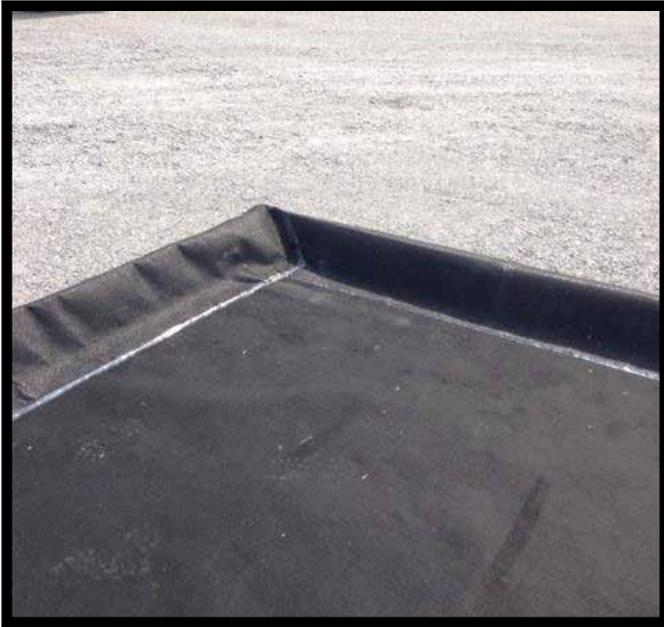
▲ Typical Padtex edge detail utilising polymer extrusion weld.
