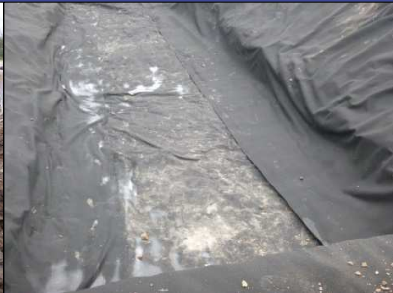
Image 2 – Lining the cell with CuTex
