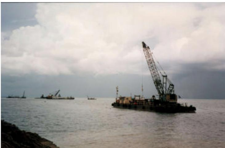
Picture 6b: Barge manoeuvring pulling the submerged roll out to sea
