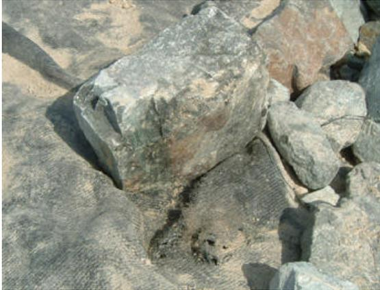
Picture 2: Damage to a woven geotextile partially constrained and small rock dumped directly onto surface causing local puncture. This could repeated many times over the whole revetment.
