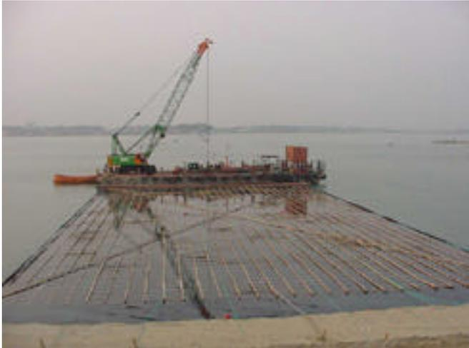
Picture 7b: Fascine mattress in and guide barge in position ready for stone dumping. The bamboos are tied at 1m centres in a latticework making the whole structure semi stiff. As the stones are placed the mattress lays down flat on the bed. The fascines have the advantage of trapping the rocks thus holding them in position and preventing them from rolling down the slope.
