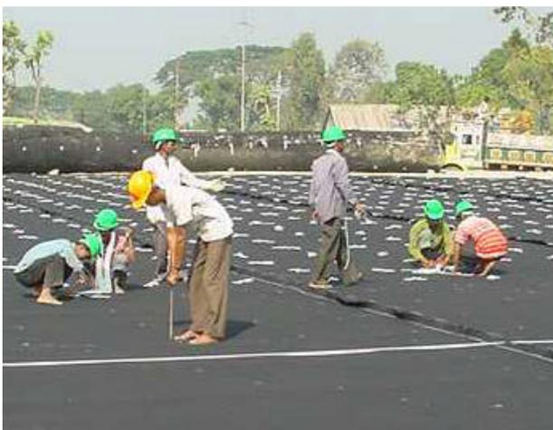
Picture 7a: Fascine mattress preparation. Note the multi width mattress approximately 25m wide sewn together. Holes are made in fabric with a push rod the same diameter as the twine used to tie fascine to fabric. Note prepared giant fabric in background.
