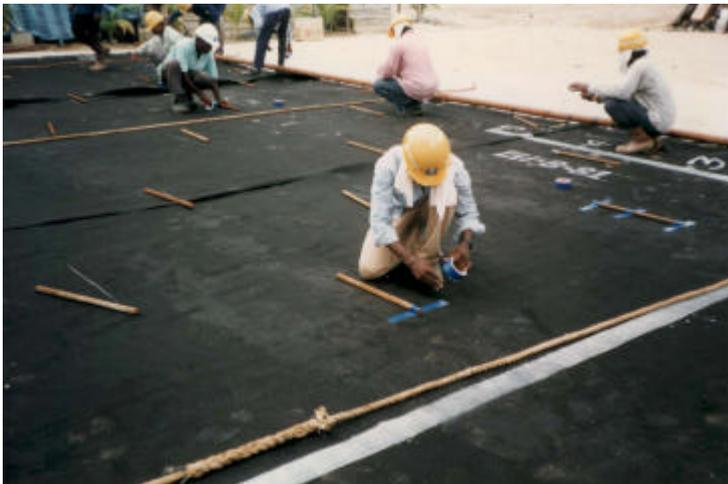
Picture 6d: Preparation of roll. Rebar being attached to fabric before being rerolled onto 12m steel bar. Note pull ropes to enable unrolling at depth.
