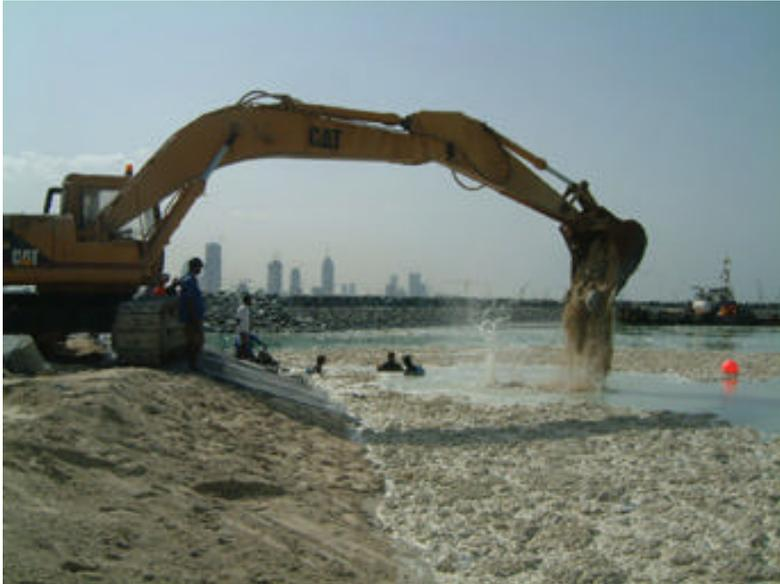
Picture 5b: Initial placement of rock to hold fabric in position. Note divers on hand to help with positioning and retrieval of pole
