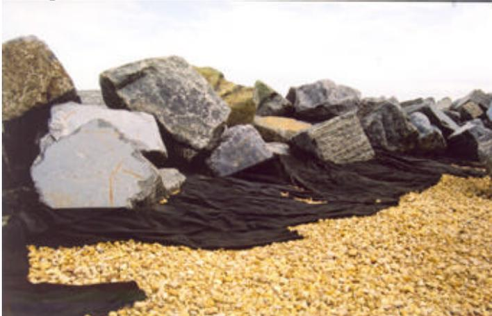
Picture 1: Damage of needle punched non woven due to high permeability 6F stone beneath geotextile instead of on top of it. Geotextile burst and tore in storm event which occurred during construction. The original design did not take into account the fact that the contractor was to build a haul road onto the beach using the Highway specification 6F material.
